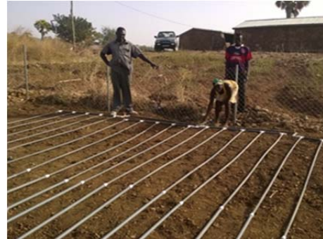
Farmer installing a drip kit designed by the University for Development Studies, Ghana. (Photo : Dr. Sylvester Ayambila, UDS)
